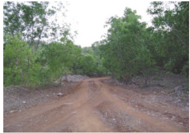
Plantation on Sides of Mining Road
